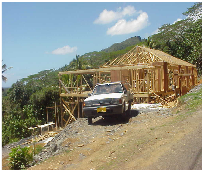
Photograph 5.0: A typical work site on sloping lands.
